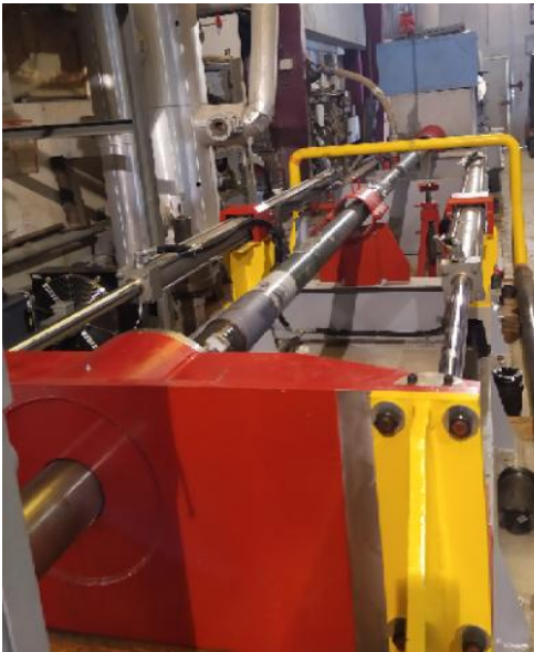
Figure 14: Horizontal Drilling Set Up
