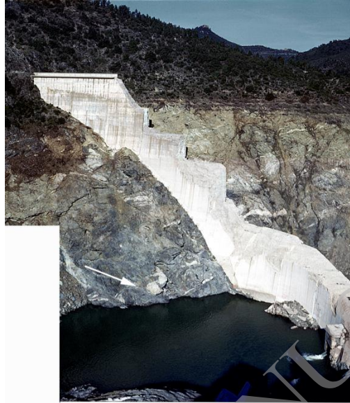
Fig. 6. Remains of the dam on right valley side and valley bottom; the rock appears crisscrossed with white pegmatite dykes; the arrow shows the main fault; the river flow passes through the outlet valve (two assembled photos, J. Duffaut, Dec.20, 1959)
