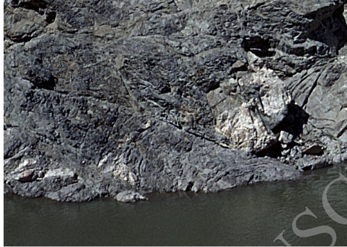
Fig. 10. Close-up on the fault cross-section at the foot of right bank; the finely crushed layers are clearly visible on both sides of the fault material (photo P. Duffaut, May 1960)
