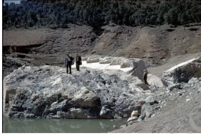
Fig. 9. The two main concrete blocks, 600 m downstream of the dam: on the one overturned, the foundation rock keeps adherent to concrete (photo J. Duffaut, 20 Dec. 1959)
