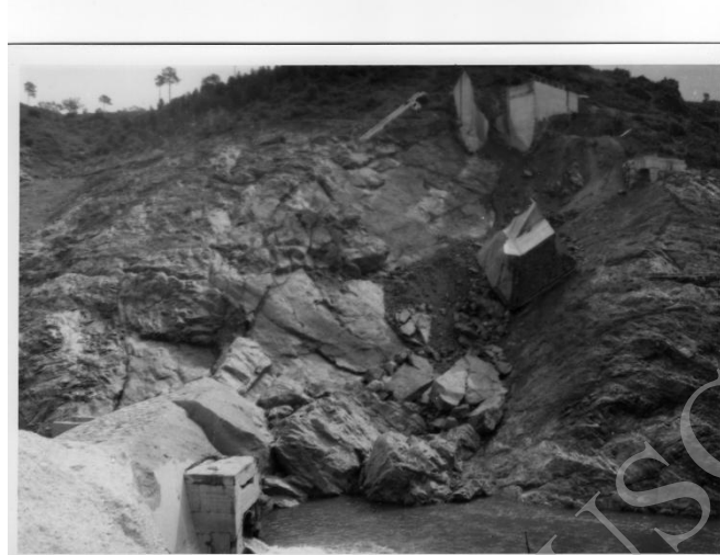
Fig. 7. The "dihedron", a deep excavation cut inside left valley side at the foot of the dam. The concrete block inside has fallen from the thrust block after the flow (photo P. Duffaut, May 1960)
