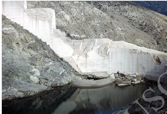
Fig. 12. The debris sill built under water by the flow below cantilever FG (photo P. Duffaut, May 1960).
