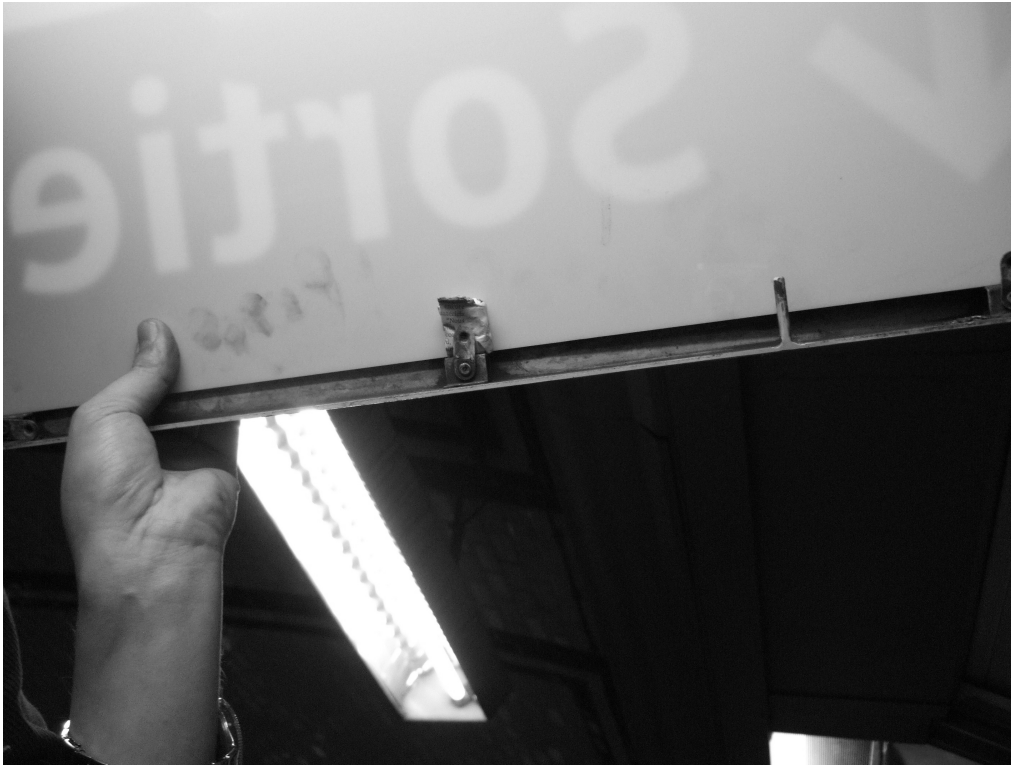
Figure 6.3. Fitting the sign into the lightbox. © Photo: Jérôme Denis and David Pontille.
