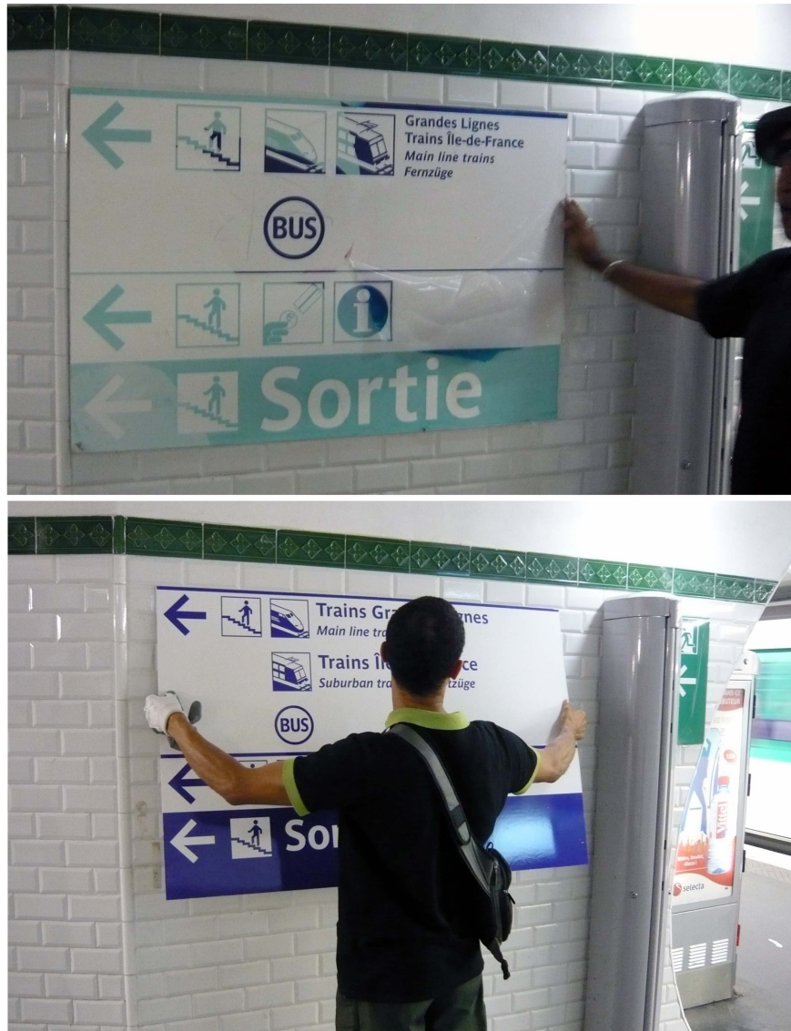
Figure 6.1. The replacement of a flawed signboard. © Photo: Jérôme Denis and David Pontille.
