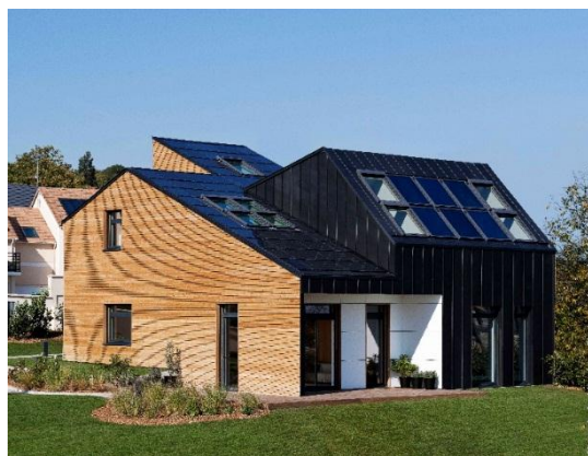
Figure 4: The nZEB Active House Maison Air et Lumière, located near Paris. © Adam Mørk
