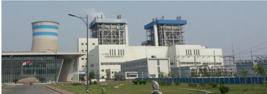
Figure 3: Tianjin Guodian coal power plant (China).
