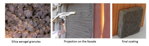
Figure 2: The new aerogel-based insulating rendering
