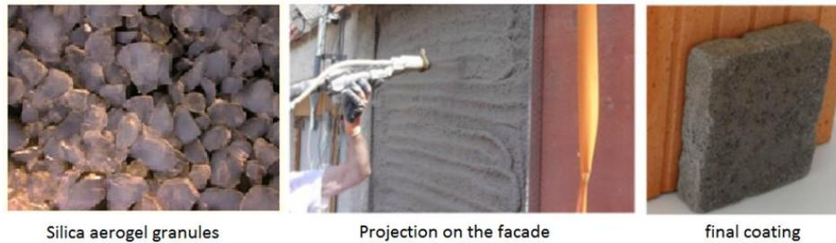
Figure 2: The new aerogel-based insulating rendering
