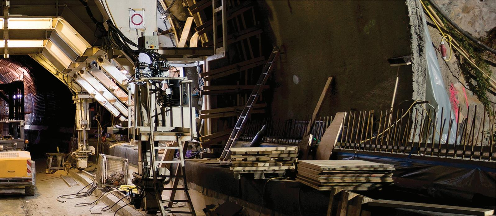
remarks were highlighted by Janin (2012): while the face bolting undergoes tension loads to improve face stability and reduce settlements, the umbrella arch mainly absorbs bending moments but does not affect surface settlements significantly.
