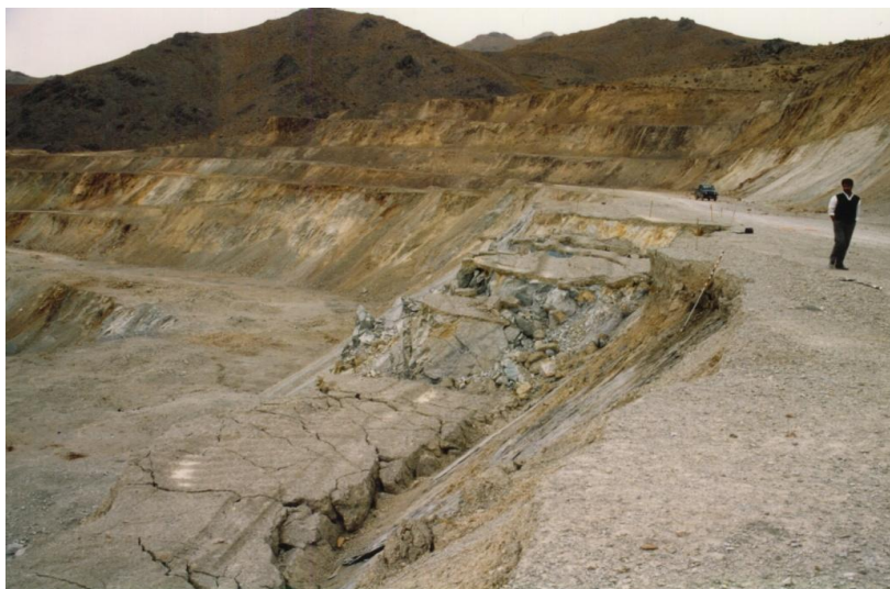
Figure 7 : South west slope of Sar Cheshmeh copper mine in Iran. Overall view and wedge failure mechanism
