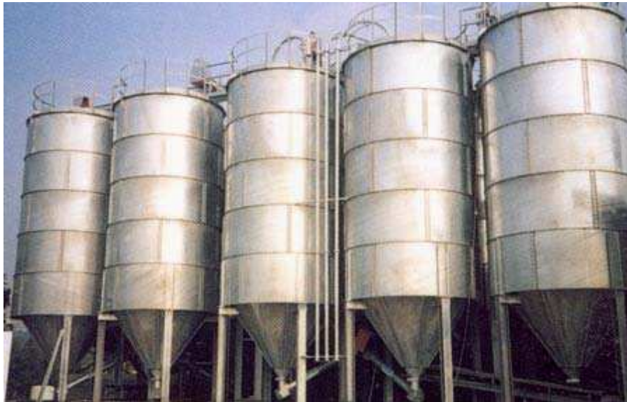
Photo 1. Examples of silos
