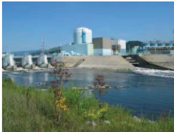
Figure 1 - Krško Nuclear Power Plant
