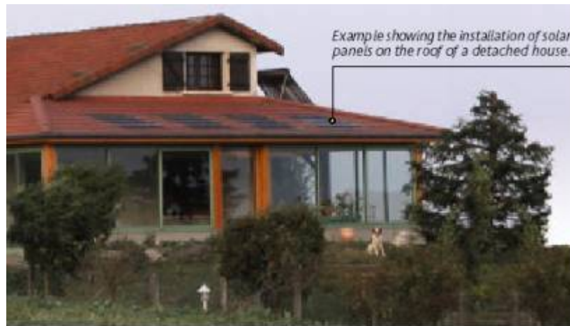
Fig. 1.13 : General overview of F1 system and of its roof integration with PV tiles.
