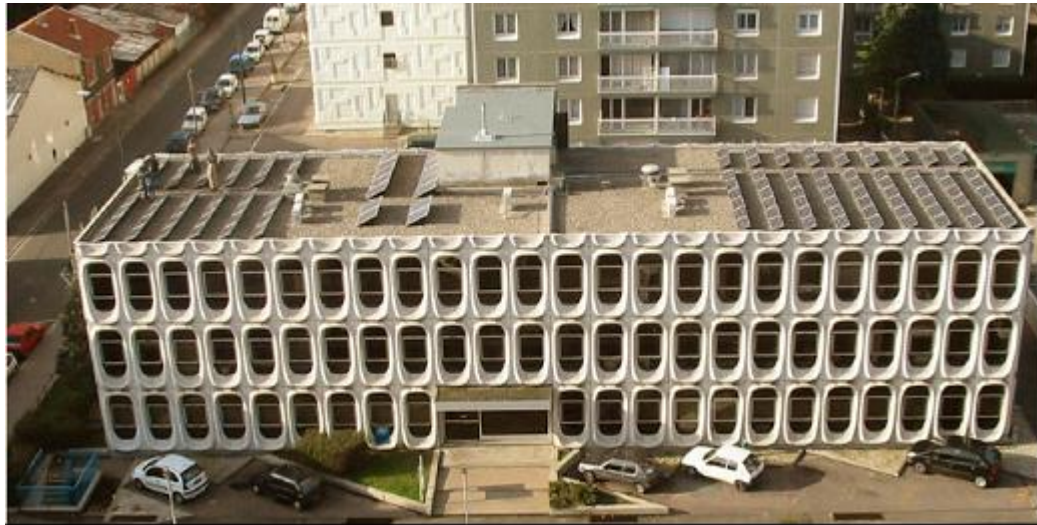
Fig. 1.6: General view of the « Soleil Marguerite » installation and of its urban environment.
