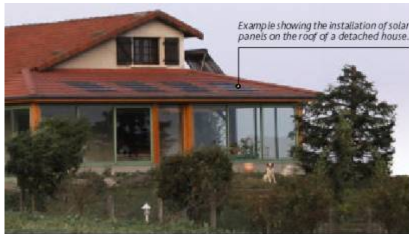
Fig. 1.13 : General overview of F1 system and of its roof integration with PV tiles.
